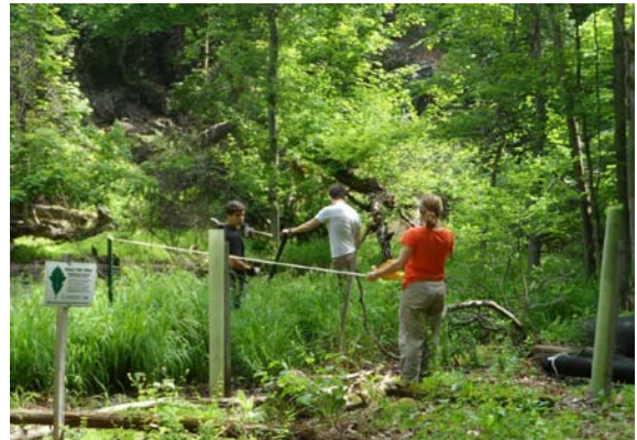
Figure 6: Pound Ridge Land Conservancy interns installing a deer-proof fence
